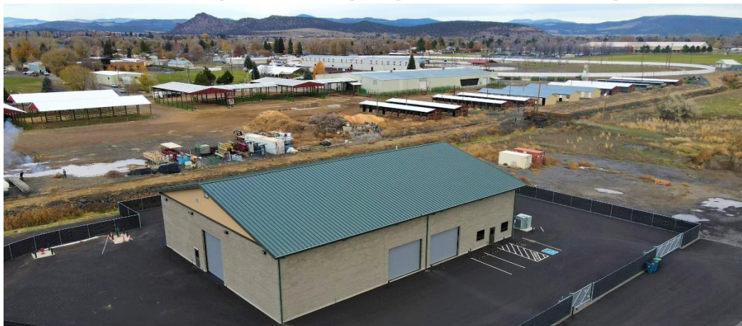
Water treatment plant facility in winter of FY 23.
