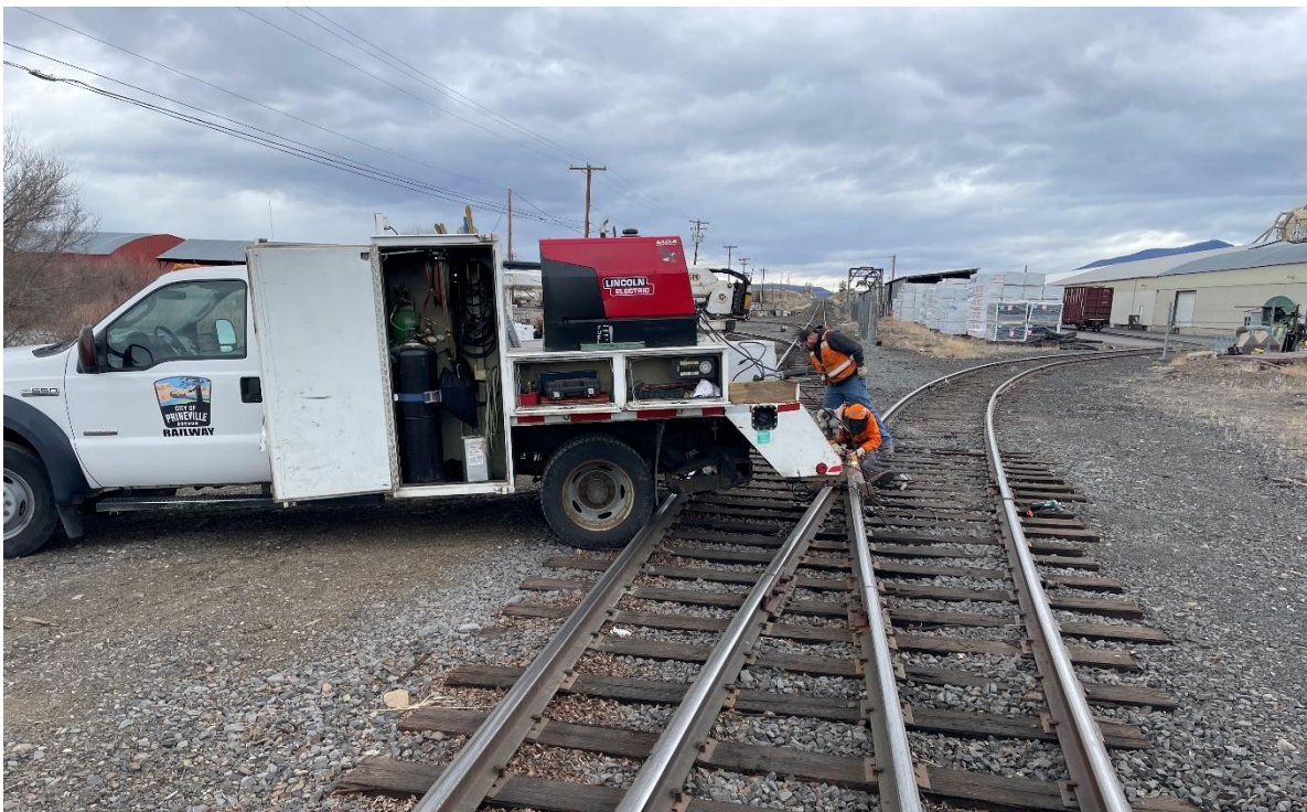
Railroad crossing work getting gone by railroad staff.
