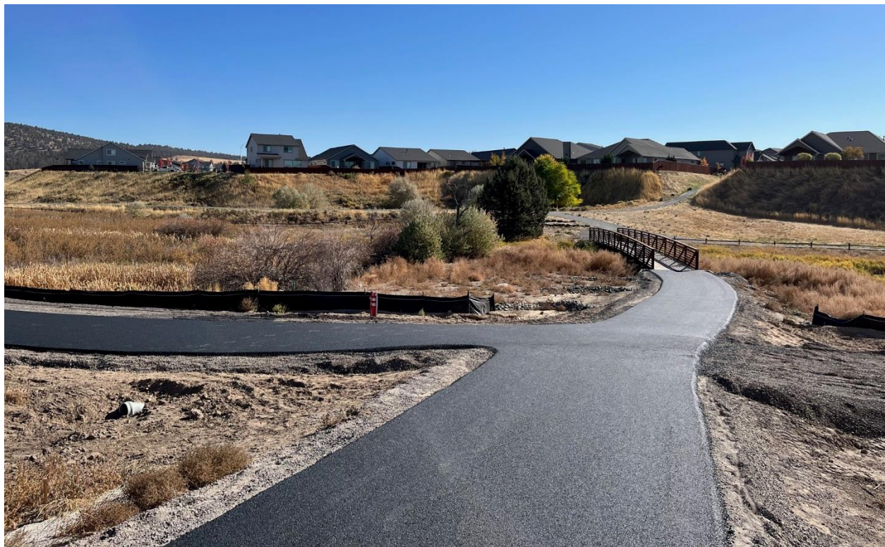
Trail paving work started at the tail end of the second quarter at Barnes Butte
