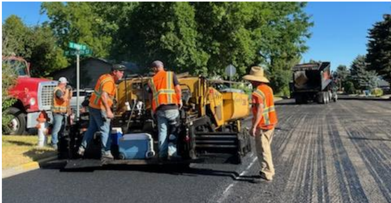
Street paving projects being done during the first quarter.
