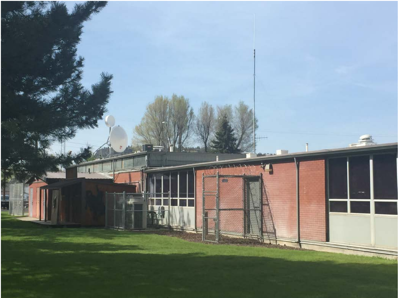
Antennas, microwave radio equipment and newer HVAC system on the exterior of the aging police department building.
