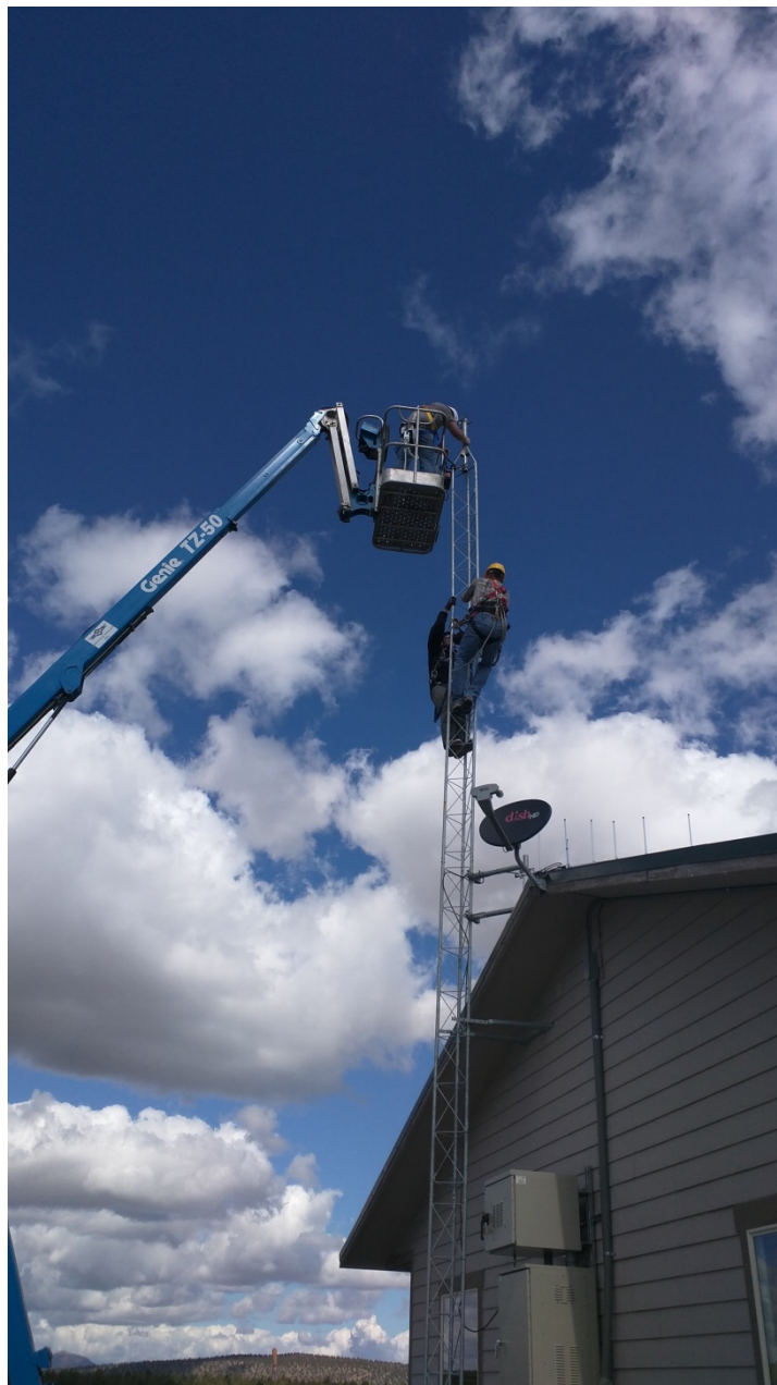
Cameras being installed at the airport by IT.
