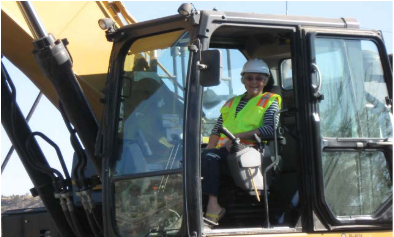
Mayor Betty Roppe helping out on a sewer installation project.
