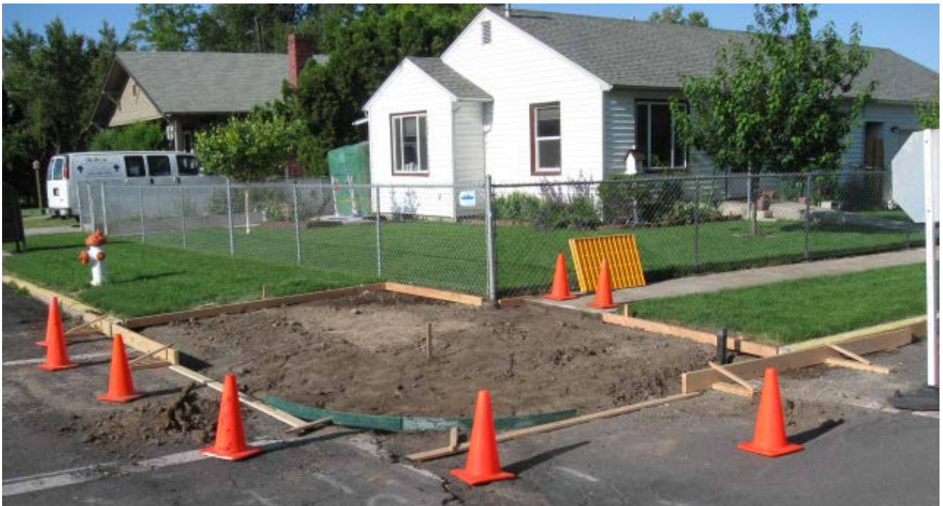
Replacing an ADA ramp near a local school
