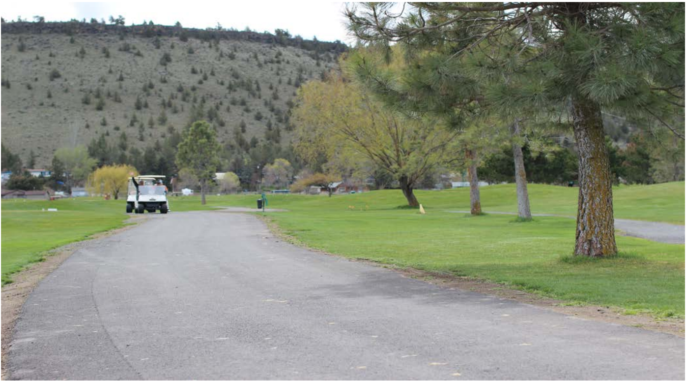
Golfers enjoying a section of newly refurbished cart path.
