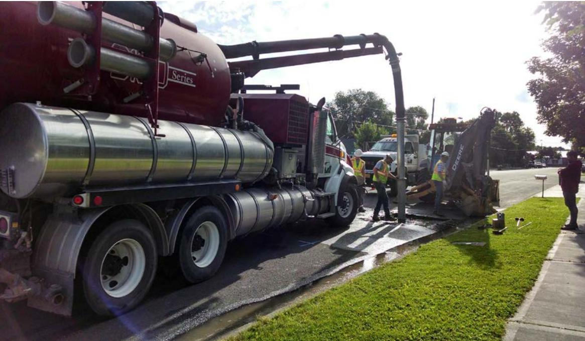
Installation of a new water service.
