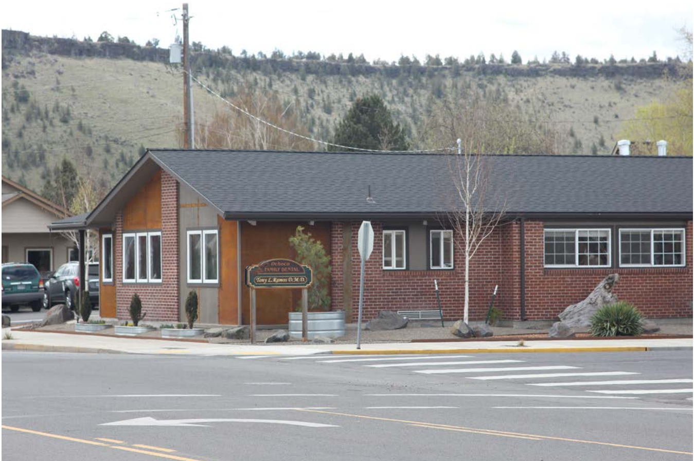
Recently renovated office of Tony Ramos D.M.D.
