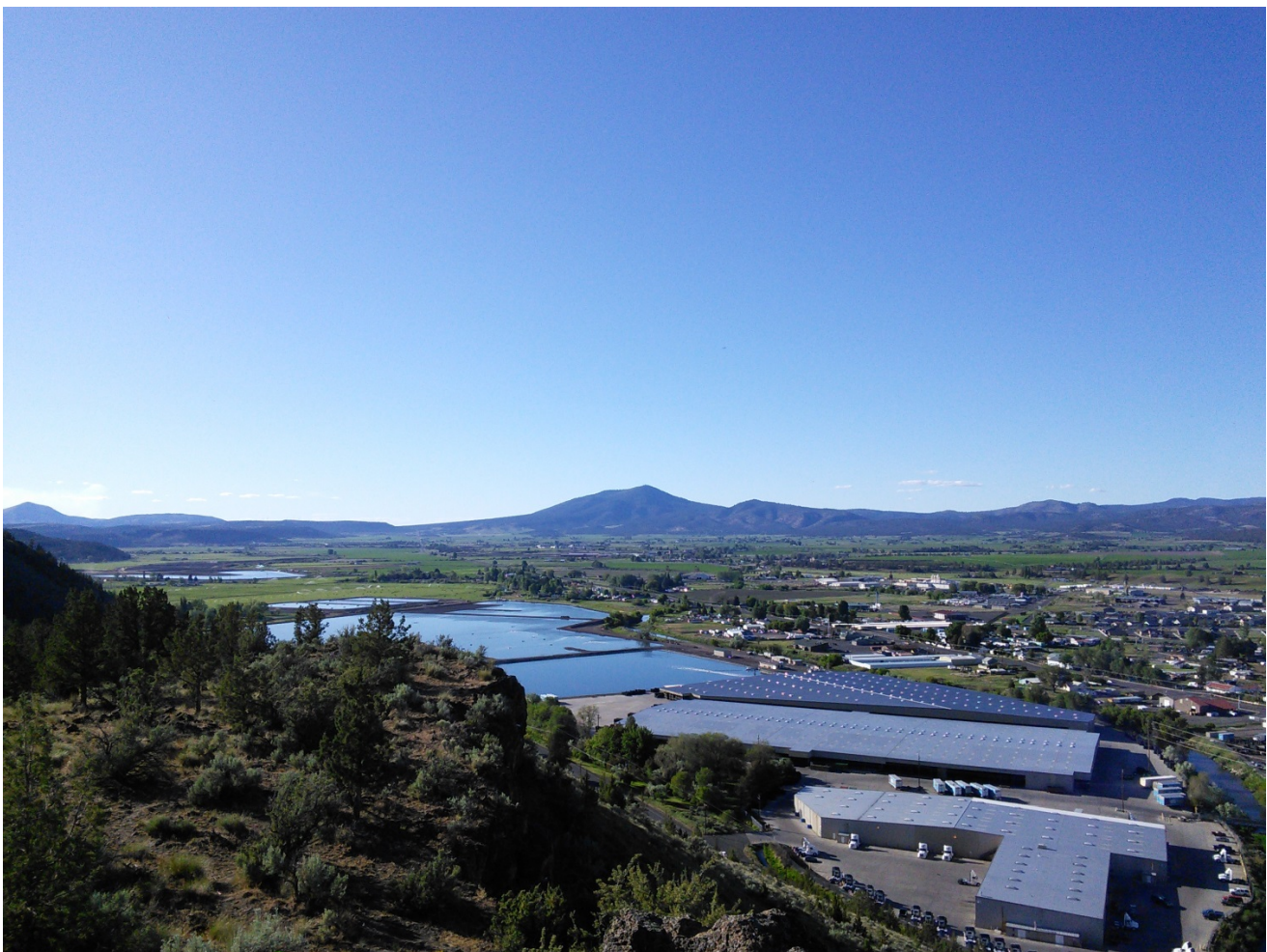
May 2016 overlooking the wastewater treatment plant ponds.
