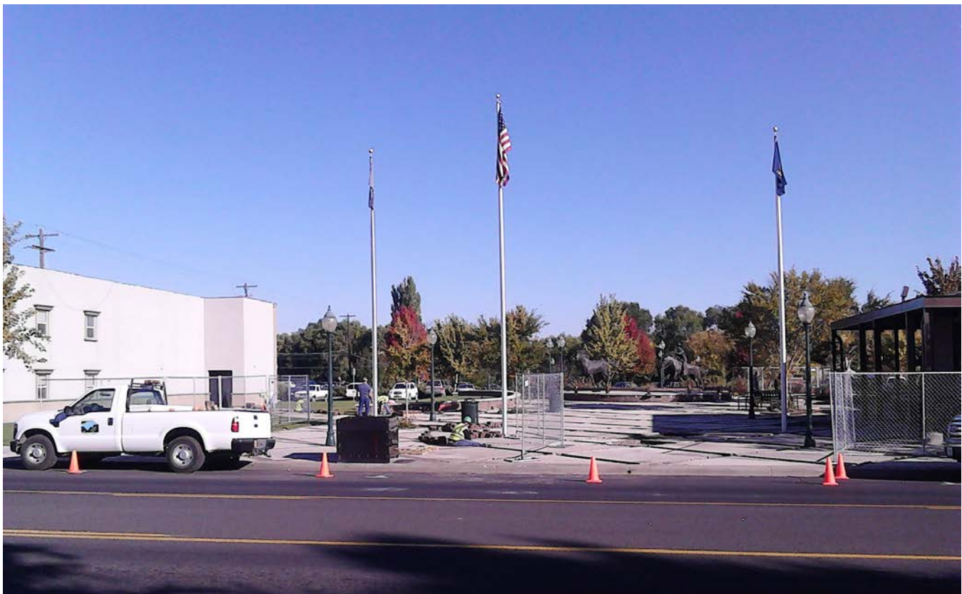
Workers remove stone pavers ahead of new concrete pour.
