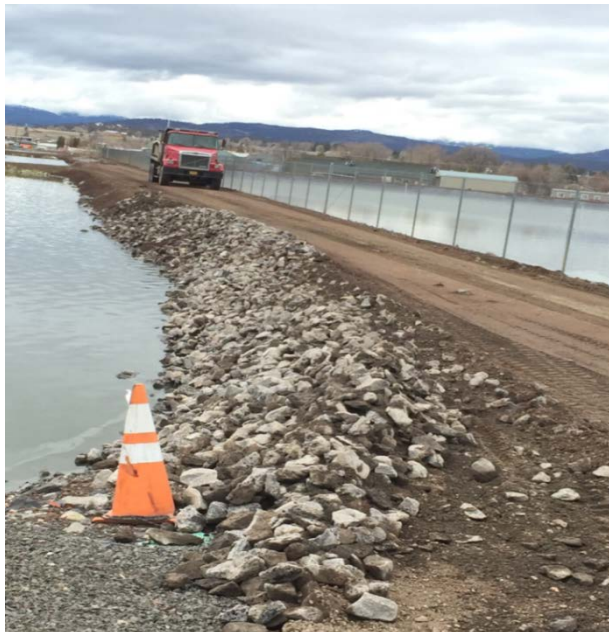
Street Department widening dikes at the Wastewater Treatment Plant
