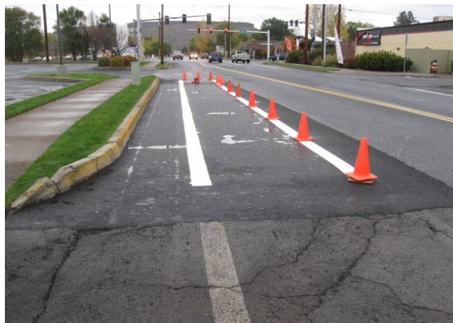
Bike Lane Restoration
