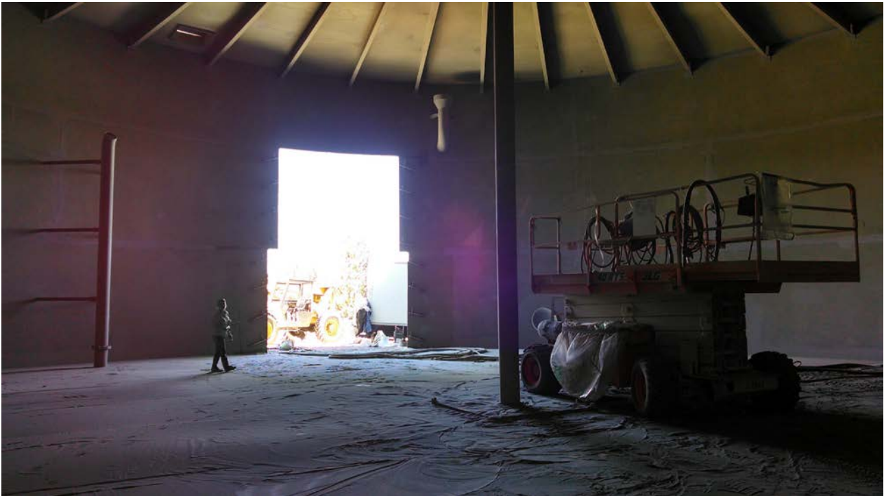
Construction progress of Airport Tank #2.
