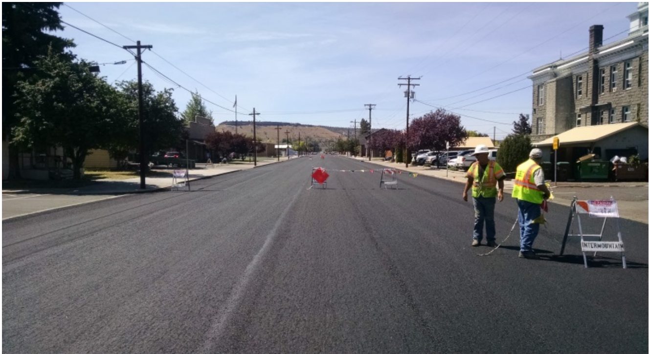
Seal coat in progress.
