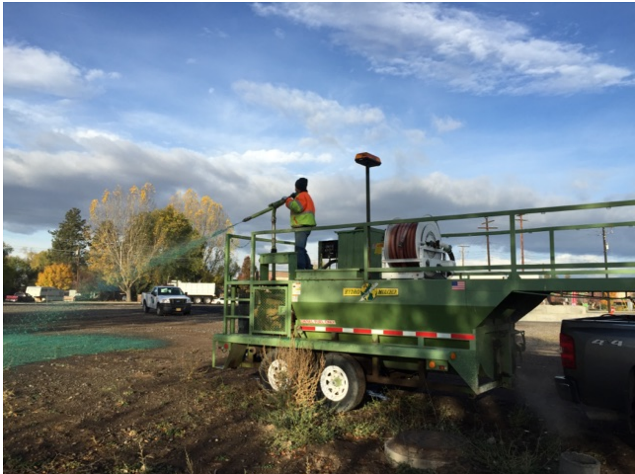
Public Works hydro-seeding.
