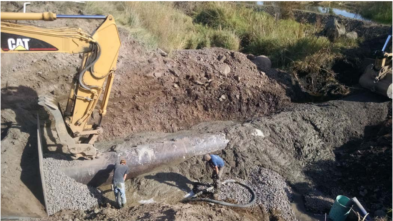
Installing main lines for new hospital site.
