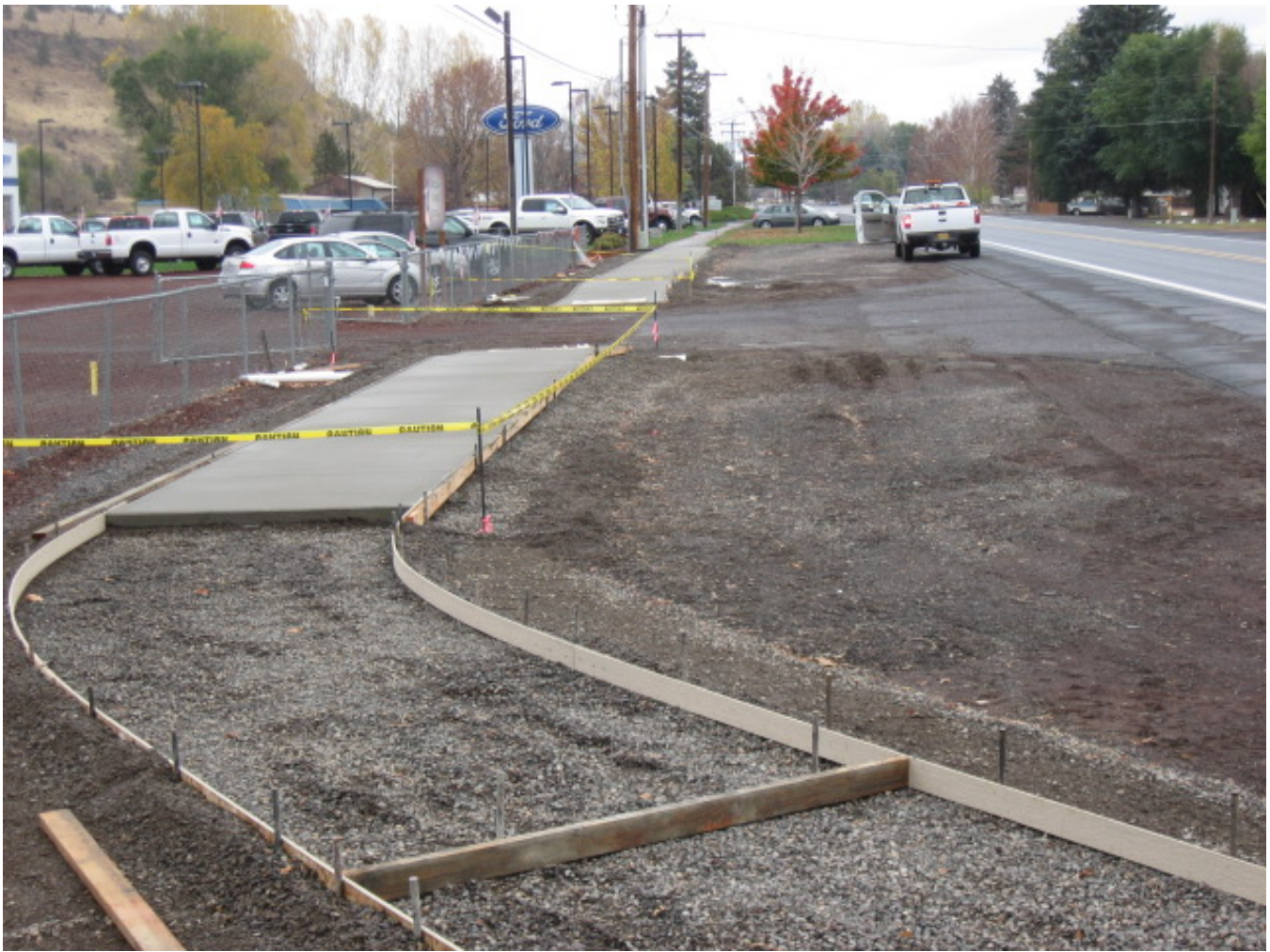
FY 16 Sidewalk infill project
