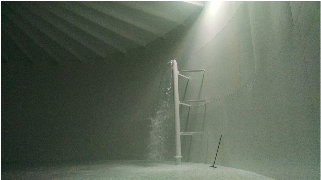
Filling Airport Tank #2 after its completion in 2014.
