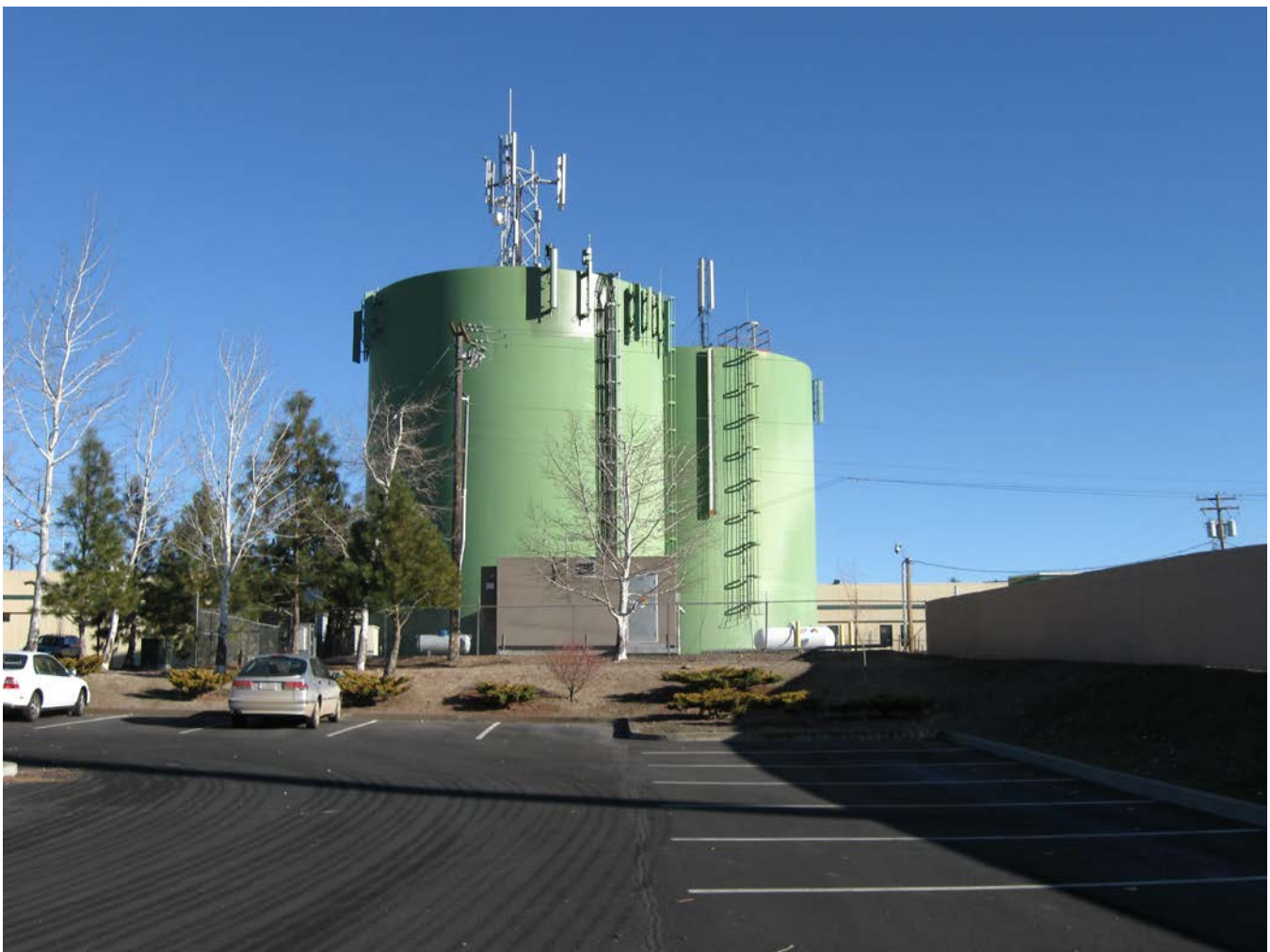
Water tanks near Pioneer Memorial Hospital.
