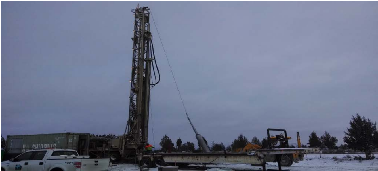
Initial drilling on Airport Well #3.
