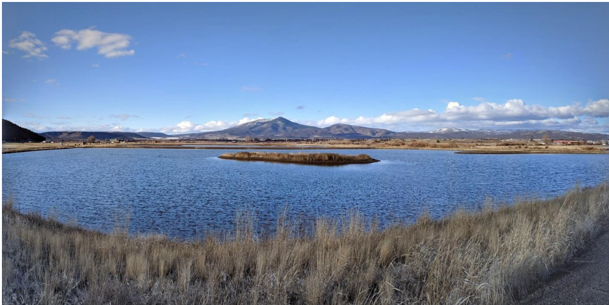
The Crooked River Wetland Complex (pictured above) is part of the City's wastewater system and accounted for in the Wastewater Fund.
