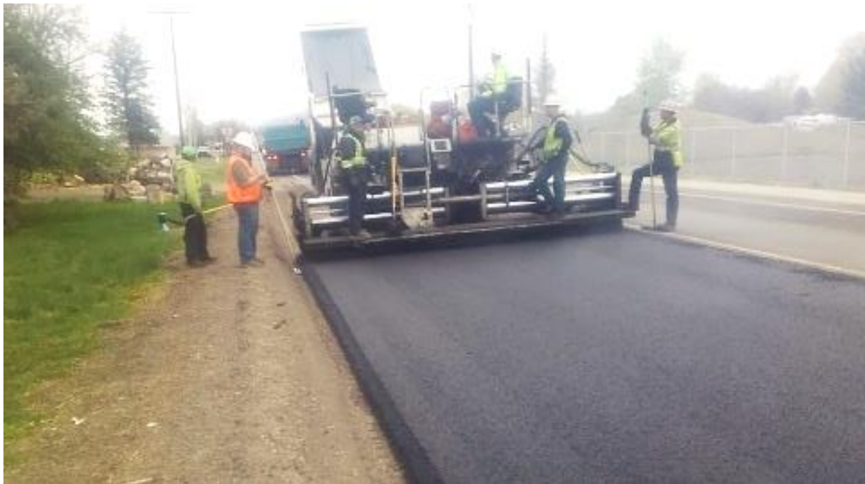
Paving on South Main that took place during the fourth quarter
