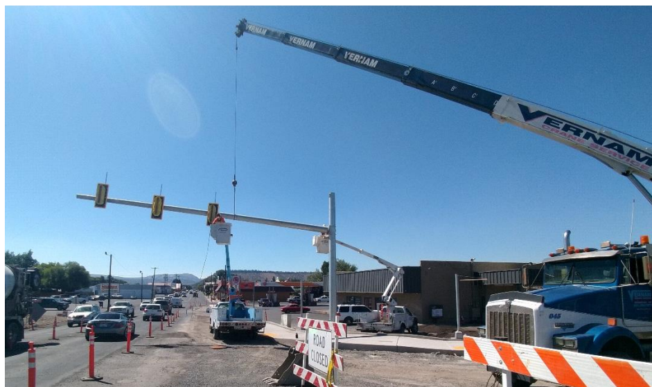
New signal being installed at 10th and Main Street in August 2021.
