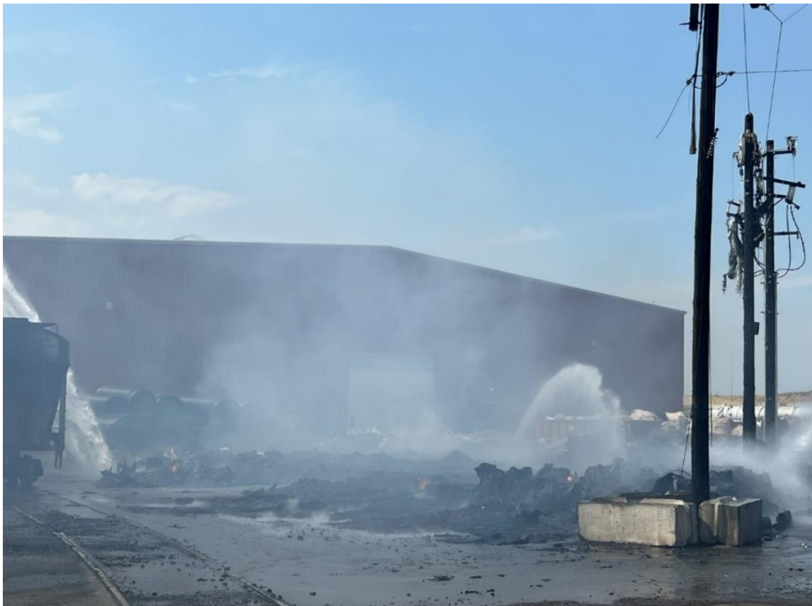
Fire being put out at the Freight Depot in August 2025
