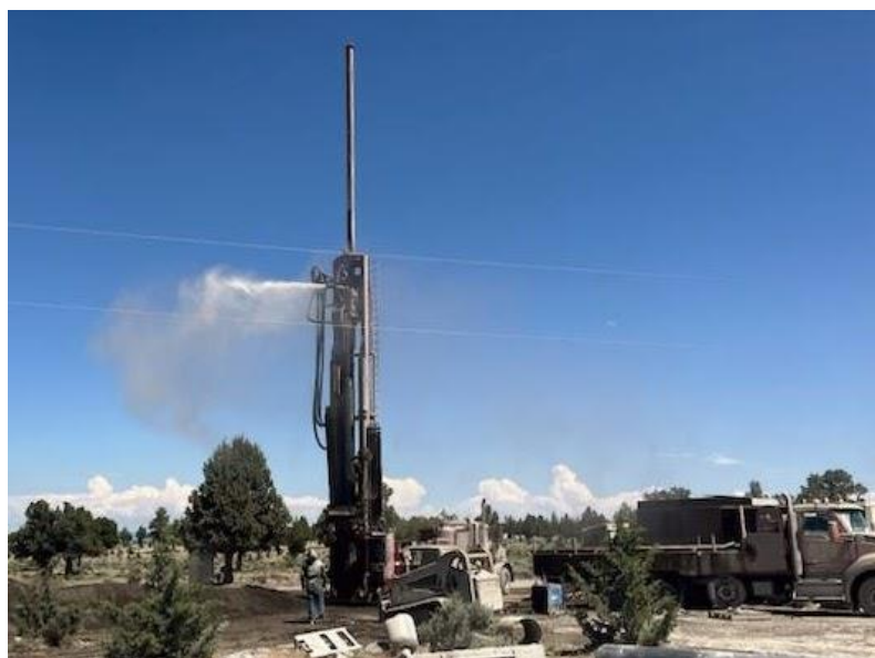
Well work being done in July 2025.
