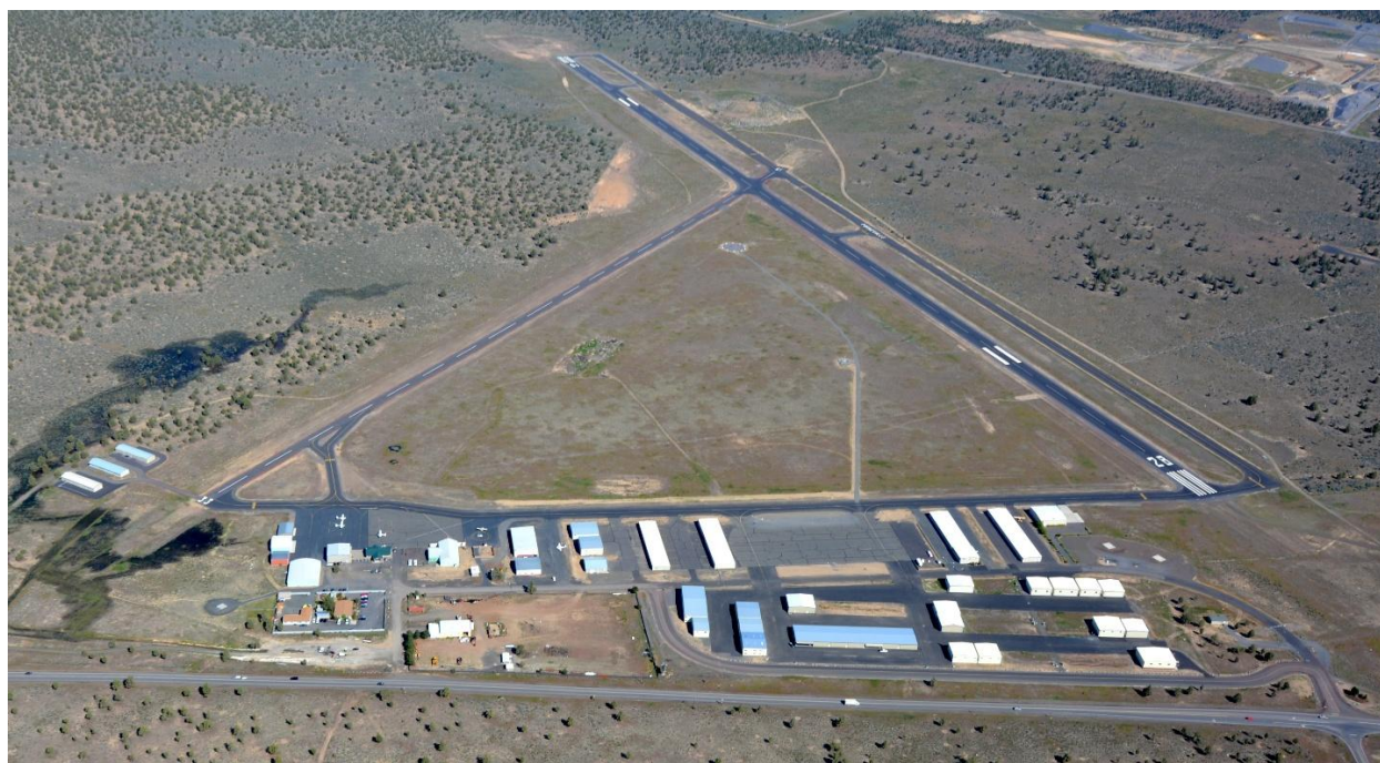
Figure 22. Prineville Airport (source: Wikimedia Commons)
