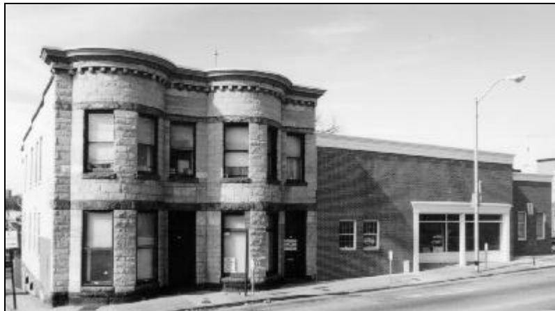
Figure xx.x This photo shows how the new infill structure on the right does not respect the existing historic architecture of the building on the left. Note how the infill structure is single story and has little or no wall articulation.
