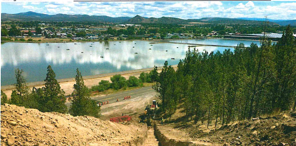
Beginning phase of the Airport Industrial Park Utility Expansion project- picture courtesy of Taylor NW
